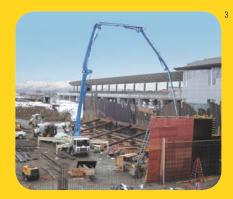
Lighter and more resilient, Putzmeister's "smart design" boom incorporates welding seams below the edge of maximum stress. The boom is engineered to offer the flexibility to adapt to different loads and features more straight pipe for a less stressful concrete flow and longer wear on parts. The Z-Fold configuration handles space restrictive areas and can pump even if the boom is not fully extended.
